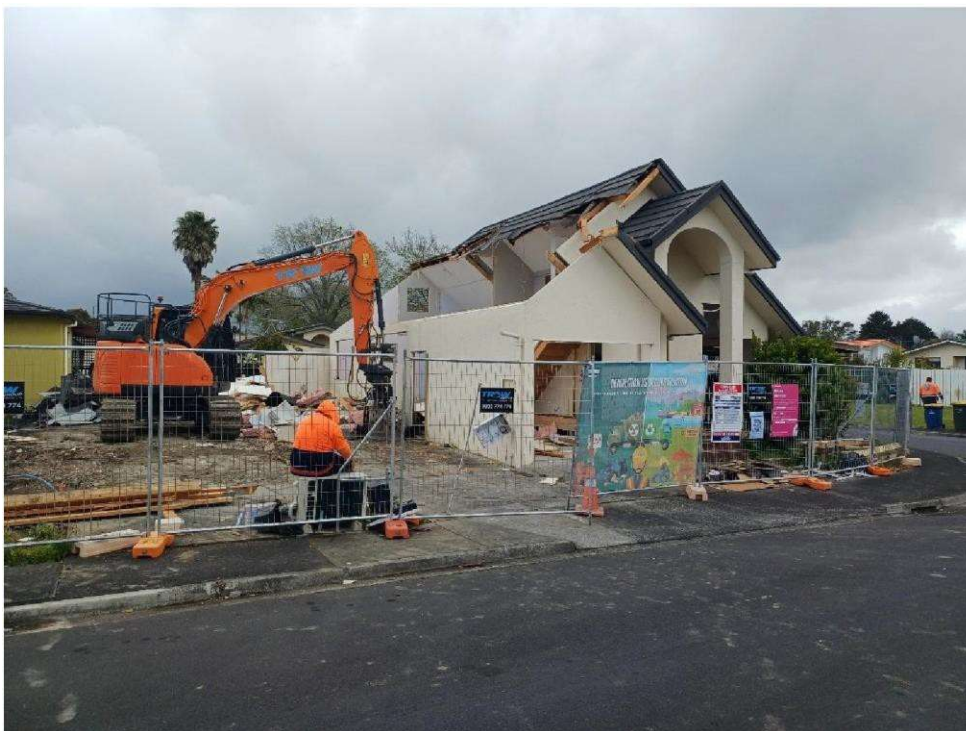
Mechanical deconstruction in action
